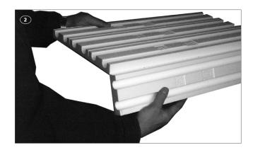
If tiles are to be laid directly on the Roth QuickTemp Compact® plates, all plates must be bonded to the subfloor. Roth QuickTemp Compact® FLEX FIX must be used for bonding. Always follow the instructions on the packaging, and if necessary use primer on the base.
